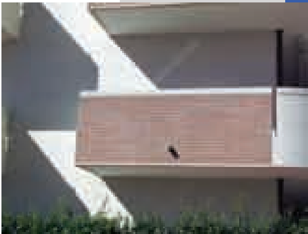
Balcons et corniches Balconies and frames
